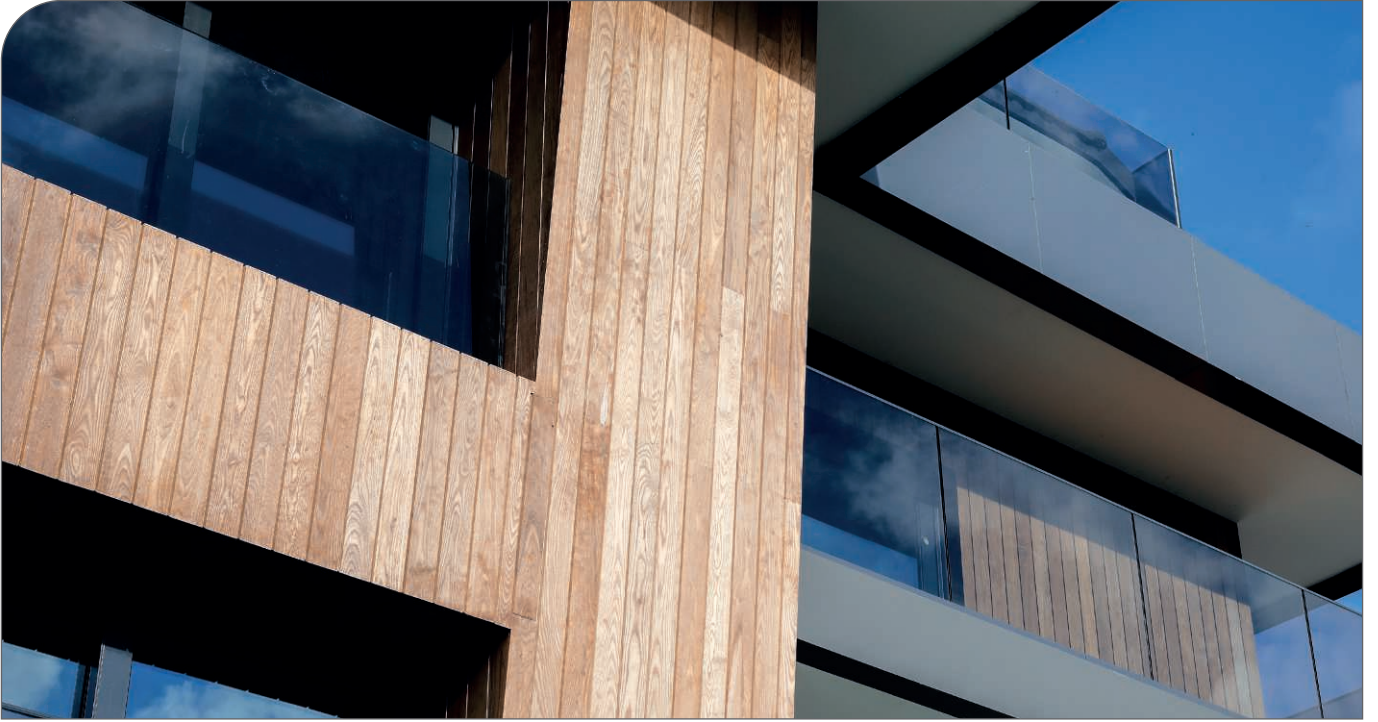
Figure 60. Exterior cladding made of ThermoWood® products. (Turkey).
