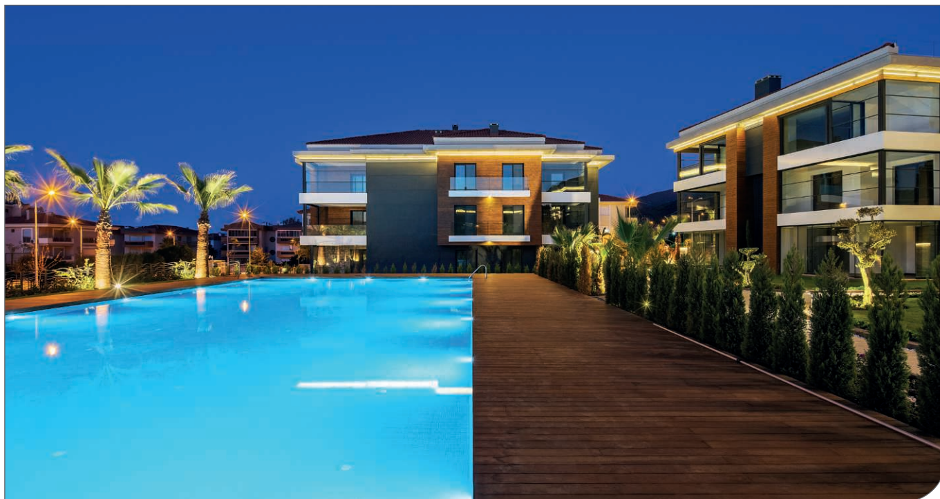
Figure 58. ThermoWood® products used for decking and exterior wall cladding on a Turkish hotel.
